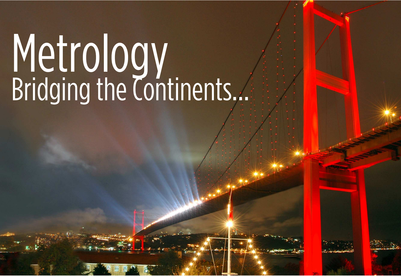
THE BOSPHORUS BRIDGE – A Gravity Anchored Suspension Bridge with Steel Pylons - (ISTANBUL 1973)
